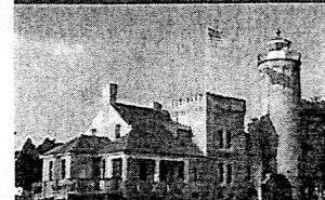
Mackinac Point Lighthouse
